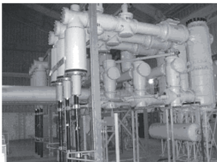
Ryc. 5. Metal-enclosed distribution board
