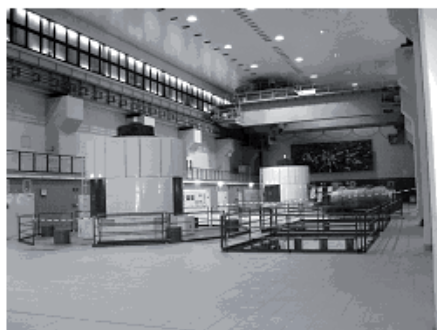
Ryc. 3. Underground cavern of turbines
