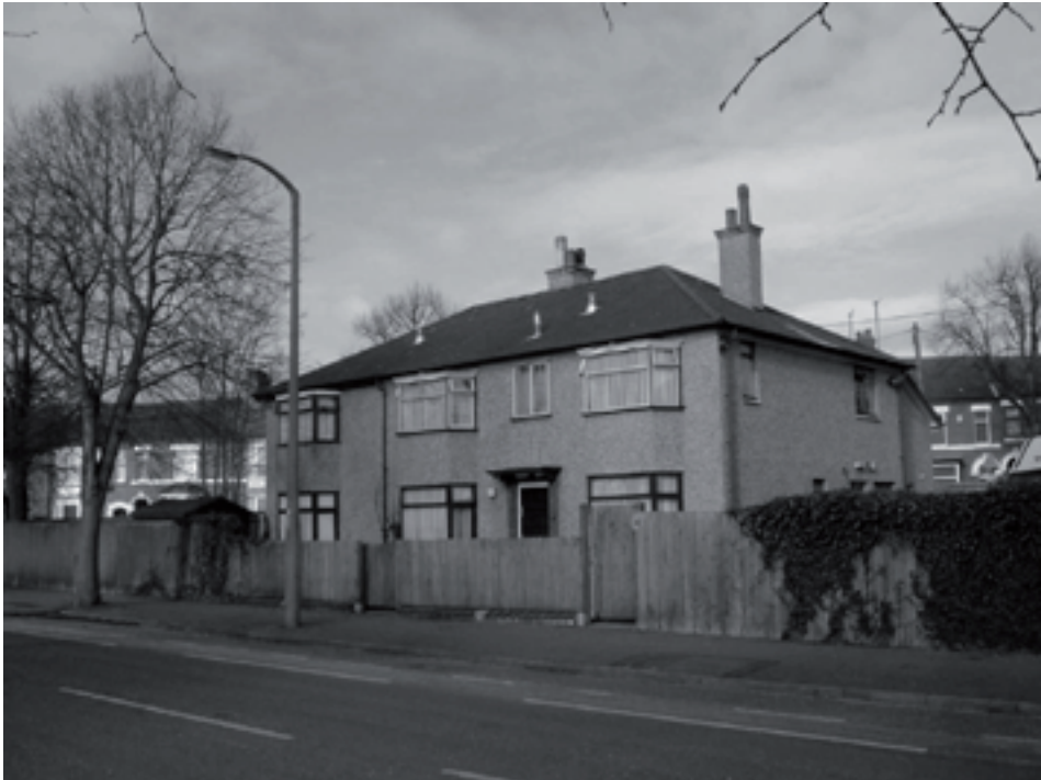
Photo 1. The residential respite care home
